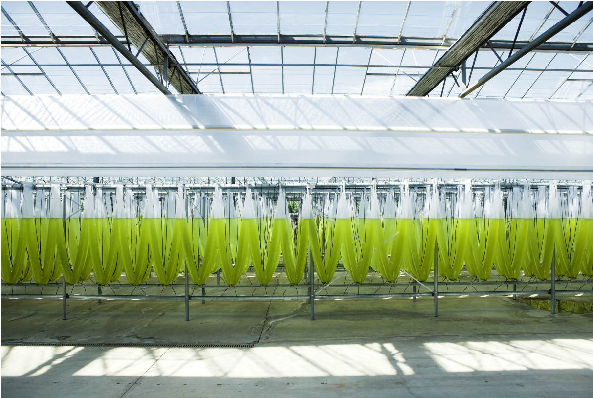
600 m 2 bioreactor at RWE coal-fired power plant
